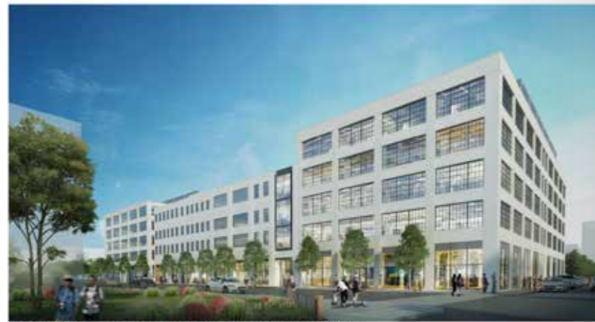
This former Polaroid building will be converted into labs and offices for startups. THE ENGINE
